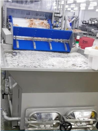
Elevated conveyor into the industrial washer
